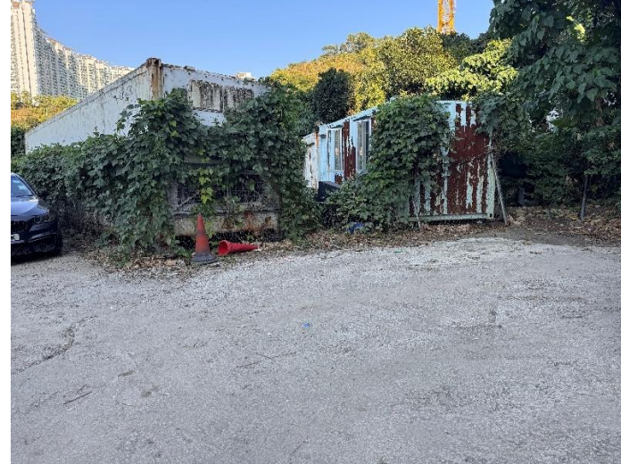
Photo 2: Storage containers are observed. However, there are no direct contact between the containers and the ground and the ground is paved with concrete in good condition. No oil stains and smells are observed.
